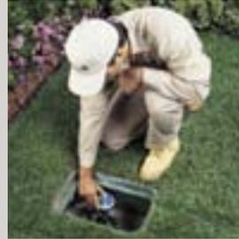
Then attach the controller to the valve (or, if it's a complete kit, install the combination controller/valve).
