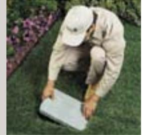
Replace the valve box cover and the hermetically-sealed controller is protected from water, dirt and contaminants.
