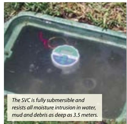
The SVC is fully submersible and resists all moisture intrusion in water, mud and debris as deep as 3.5 meters.
